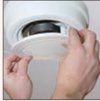
3. Snap the grille into the mounting ring.
