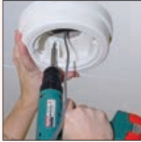
1. Fit the surface mounting ring.
